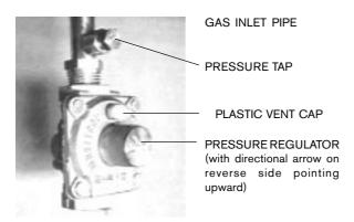
Fig. 5 - Installation of Gas Pressure Regulator
