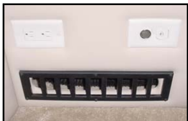
Figure 7-9. 120 VAC Receptacle
