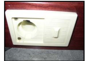
Figure 14-13. Vacuum Hose Coupling
