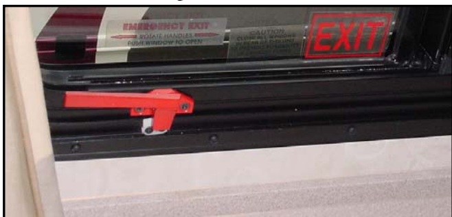
Figure 13-2. Bedroom Emergency Exit Window
