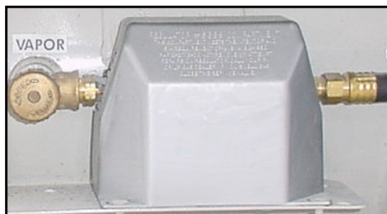
Figure 3-5. LP Gas Regulator
