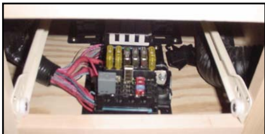
Figure 7-18. Fuse Blocks within Center Console
