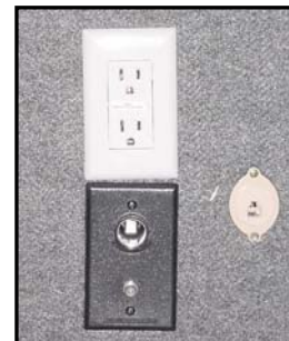
Figure 7-10. 12 VDC Receptacle (black)
