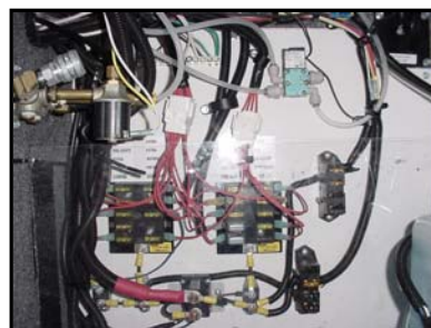
Figure 7-2. Fuse Panel
